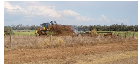
Pile burning, dozer pushing
